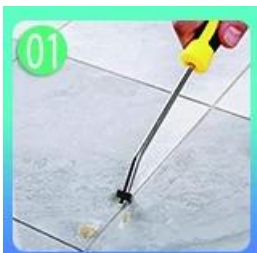
01 Clean the tiles and keep it dry
