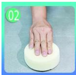
02 Polish with tile wax except the glazed tile
